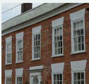
Camber flat arched render lintel above windows on the Horsford Hall facade
